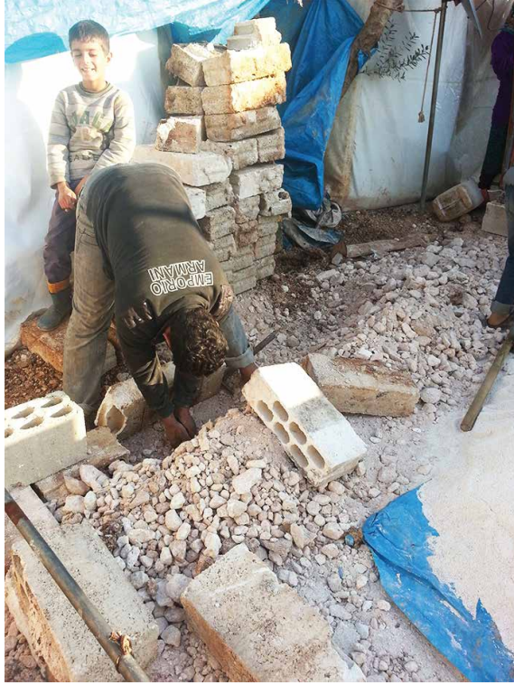
Building a Room in Al Arbayeen camp within Al Rahma cluster
