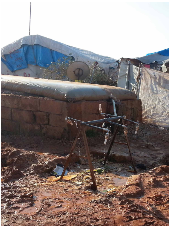
Water point in Ehsas camp within Atma cluster
