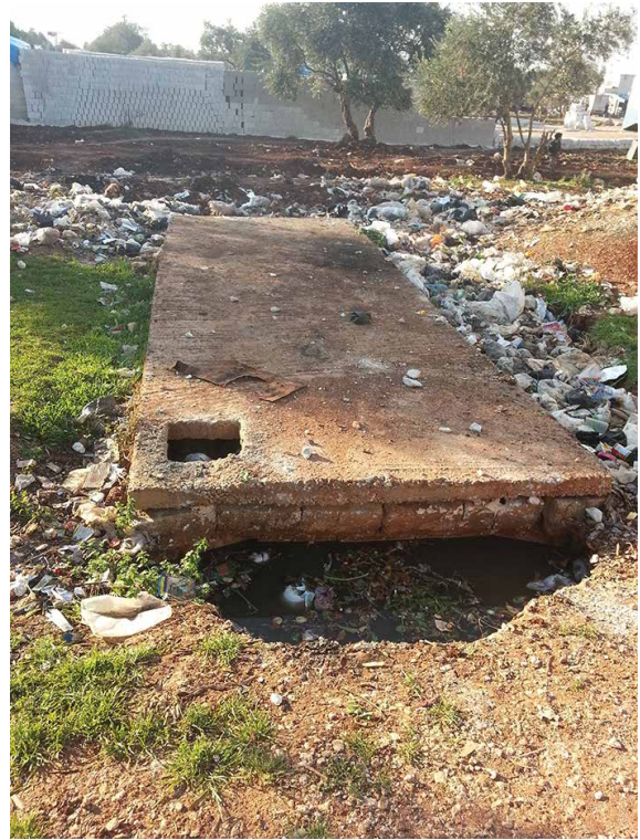
Open sewage hole in Ahbab Al Rasoul camp within Al Rahma cluster
