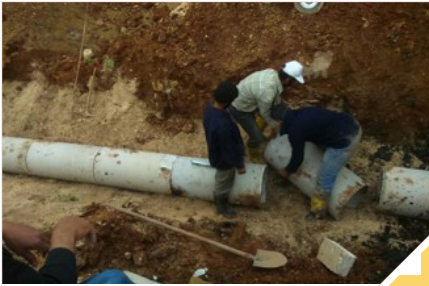
➤ Figure 69: Maintenance of water network in Belyoun _July 2019
