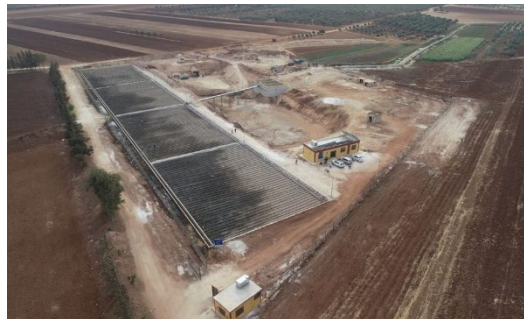
Figure 132: Ram Hamdan wastewater treatment
